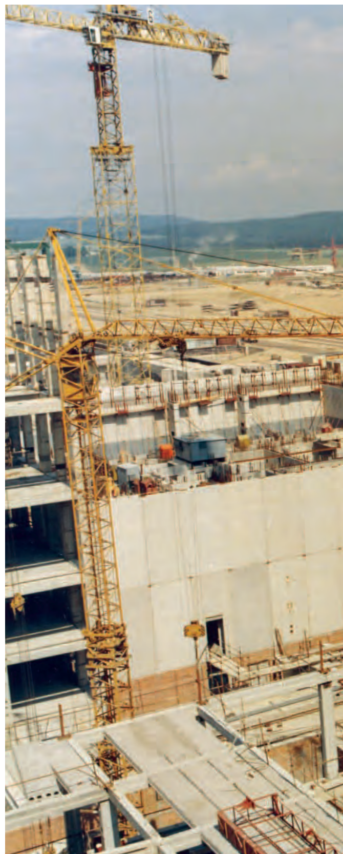
POHLED DO BUDOVY REAKTORU PŘI MONTÁŽI OBESTAVBY REAKTORU VIEW INTO THE REACTOR BUILDING DURING CONSTRUCTION OF THE CONTAINMENT ENCLOSURE OF THE REACTOR
