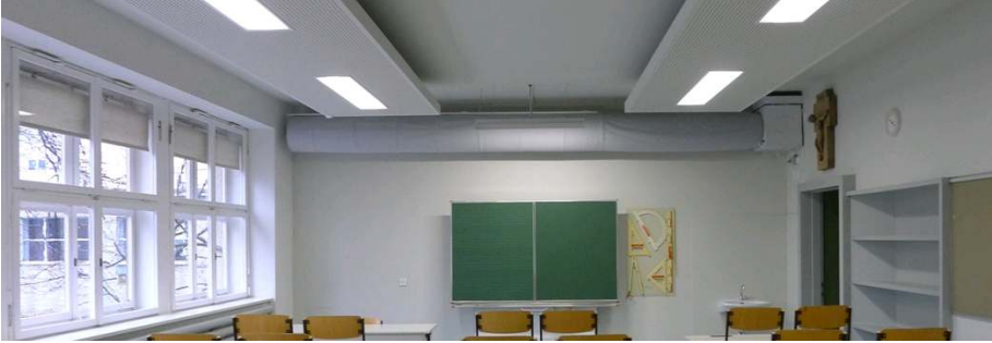
Figure 1: Silencer and fan-box prototype manufactured by ATREA
