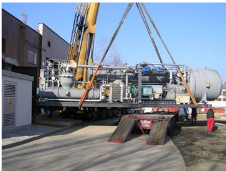
Obr.5 - Instalace modulu ORC
