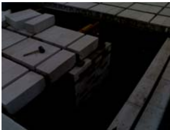
Obr. 5 Strop YTONG
